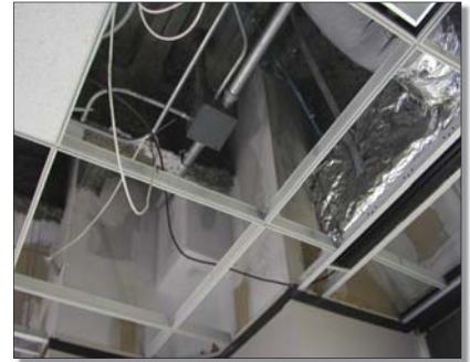
Photograph 1 (left): The Ubiquitous Dropped Ceiling Return Plenum. Who knows what evil lurks hidden above the ceiling tile? The building scientist knows. Photograph 2: Lack of Closure. The gypsum board does not extend to the underside of the floor assembly above. Note the discolored insulation due to the filtration effect of dust being retained as exterior air is pulled through insulation into the return plenum. Photograph 3: Retrofit of Closure. Gypsum board extended to underside of floor assembly and sealed, creating closure.
