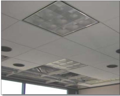
Photograph 1 (left): The Ubiquitous Dropped Ceiling Return Plenum. Who knows what evil lurks hidden above the ceiling tile? The building scientist knows. Photograph 2: Lack of Closure. The gypsum board does not extend to the underside of the floor assembly above. Note the discolored insulation due to the filtration effect of dust being retained as exterior air is pulled through insulation into the return plenum. Photograph 3: Retrofit of Closure. Gypsum board extended to underside of floor assembly and sealed, creating closure.
