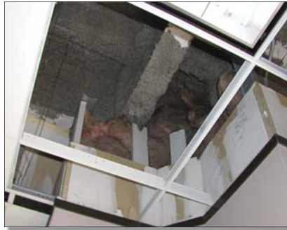
Photograph 1 (left): The Ubiquitous Dropped Ceiling Return Plenum. Who knows what evil lurks hidden above the ceiling tile? The building scientist knows. Photograph 2: Lack of Closure. The gypsum board does not extend to the underside of the floor assembly above. Note the discolored insulation due to the filtration effect of dust being retained as exterior air is pulled through insulation into the return plenum. Photograph 3: Retrofit of Closure. Gypsum board extended to underside of floor assembly and sealed, creating closure.
